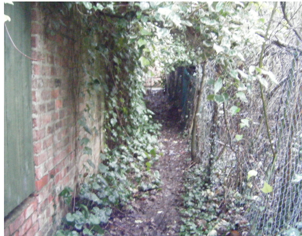
Photo 4 Narrow and overgrown section
